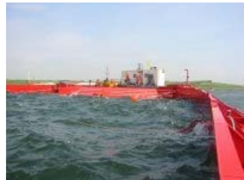
Figure 2: (Left) Basic diagram showing the function of the Wave Dragon. (Right) Picture of the Wave Dragon prototype being tested at the Danish Wave Energy Test Station in Nisum Bredning. http://www.wavedragon.net/technology/prototype.htm
