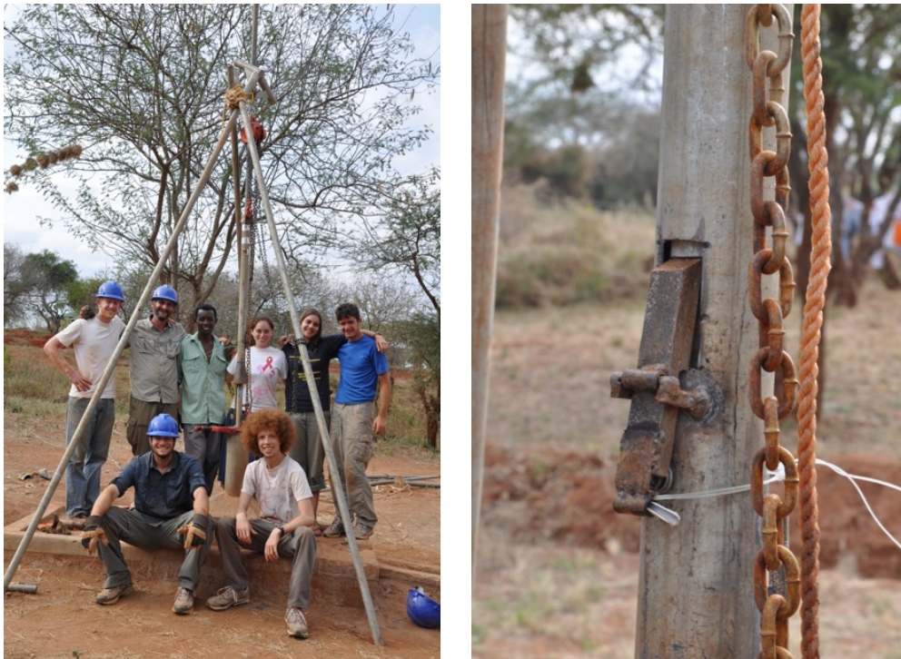
Figure 14: The Rocket emerges from the well, pipe firmly in tow. [July 10]
