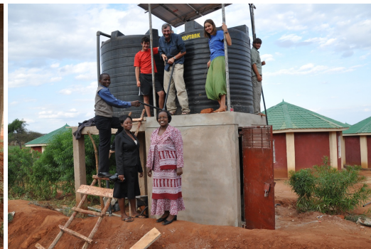
(b) The finished powerhouse, with tank and solar panels on top. We're finishing the water line into the tank from the pump. [July 13]
