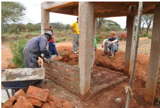
(a) Laying brick for the walls. [July 6]
